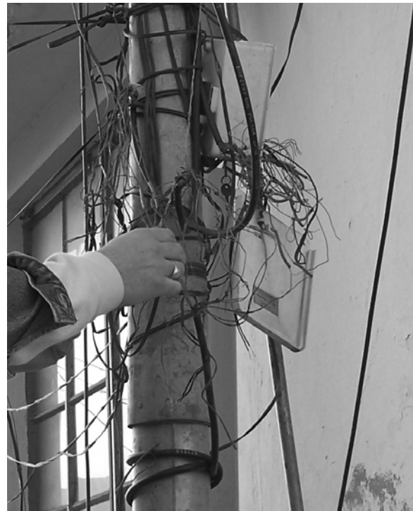
Picture 2 Troubleshooting a Telephone D-Mark
